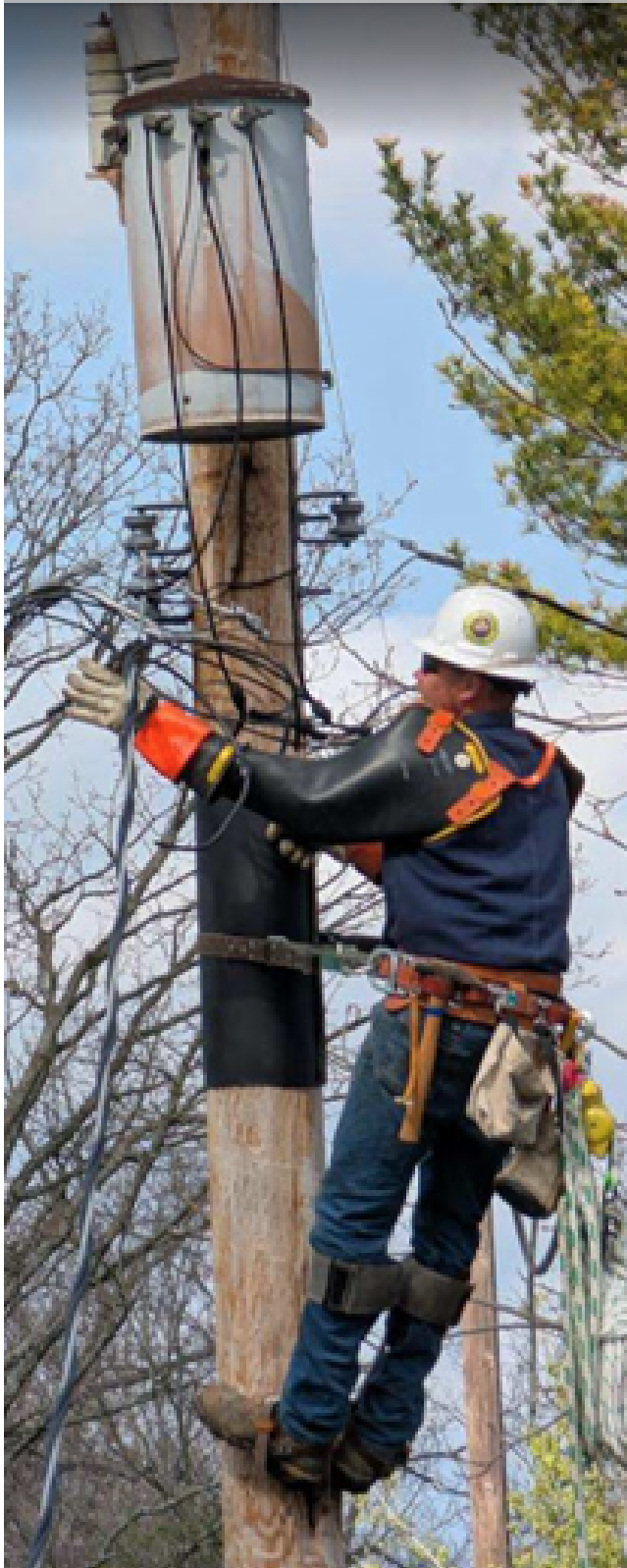
Recent electric department projects.
